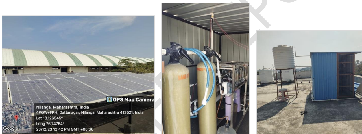
Plate 2: Investigation of the system
