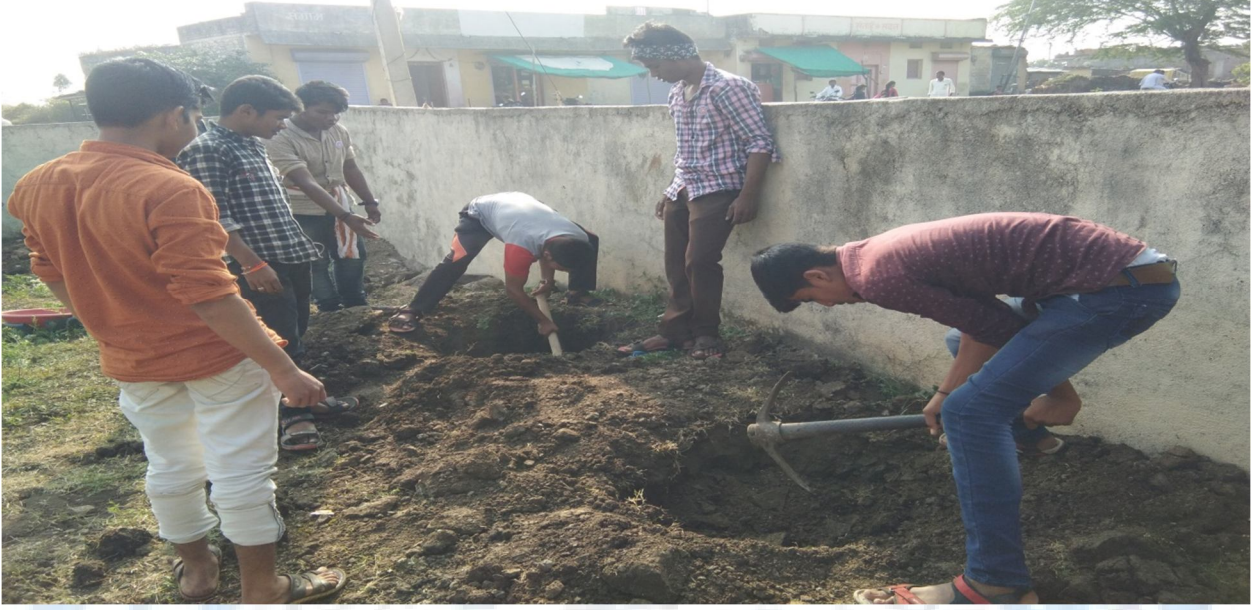
Volunteers of National Service Scheme digging ditches for sanitation
