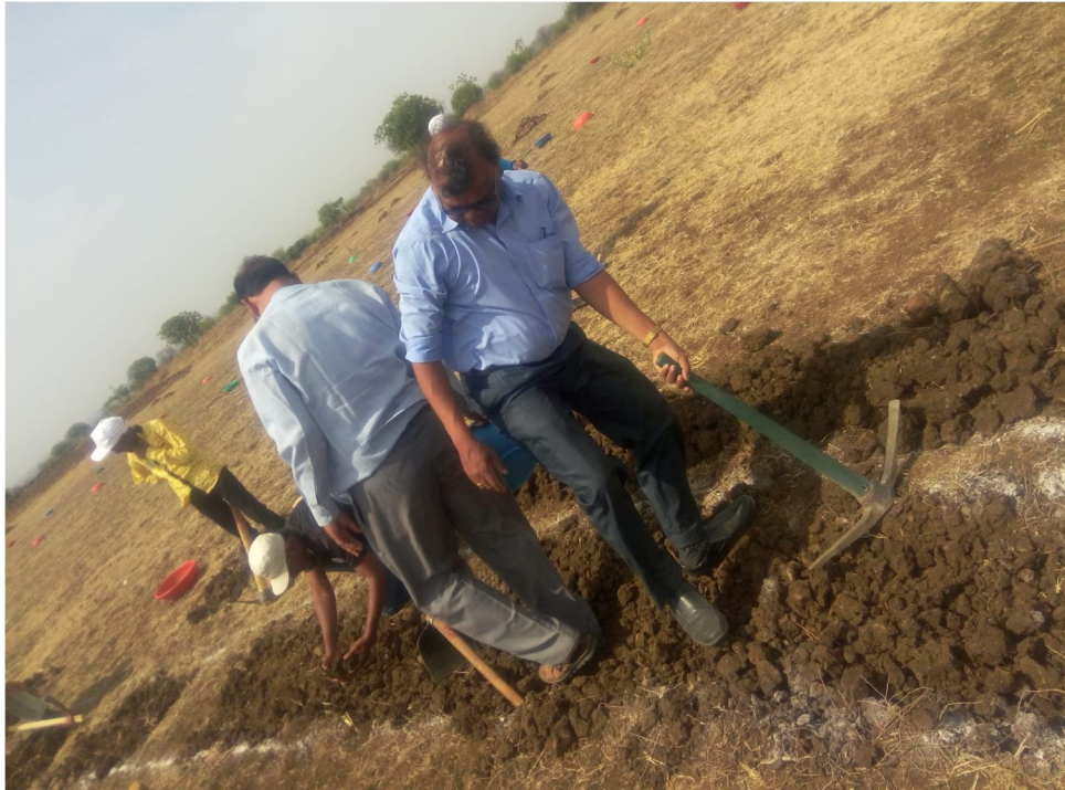
Faculties while working on the field for creating water grids
